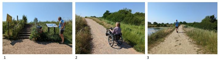
Access to the coastal path: at the start point, alongside an information board, there is both stepped access (1) with metal handrail to both sides, and ramped access with a medium gradient of approx. 1:12-15 m(?) to the sea wall. The ramp and sea-wall path is hard-surfaced (hoggin), with a dusting of light gravel.
