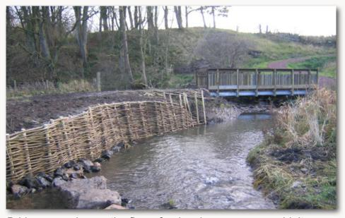
Bridges can change the flow of a river in ways you wouldn't expect. Here, the burn washed out the bank in a freak storm after the bridge was built. Have a close look at the area of willow and you'll see that we've reinforced the bank to stop the erosion, using a traditional technique called spiling: willow stems planted into the bank have been woven like a basket to hold the bank together. The bank becomes stronger, like a living wall, while allowing the water to flow over in a real spate.
