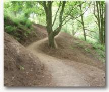
In some places the path had to be built up on an embankment of earth up to 1.5m high, in others the bank was reshaped dramatically. But the point is, it looks good. Path construction is an art as well as a technique.
