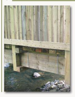
The main beams – the parts that span the river – are the most expensive part of a bridge and must last as long as possible. If you look carefully, you will see there are no bolts through these beams – anywhere. Any holes drilled for bolts would encourage rot and shorten the beams' life. This bridge design makes it easy to replace just the deck, balustrade and handrails when they wear out: much cheaper than building an entirely new bridge.
