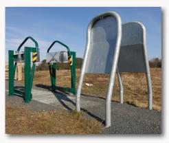
Keeping motorbikes out of places where they have no right of access is always a tricky challenge. These robust structures can help to make a point and will deter some motorbike riders, but they never solve the problem completely and horses just can't get through.
