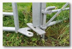
An ingenious hinge and bolt arrangement allows this gate to 'fold' in the middle.
